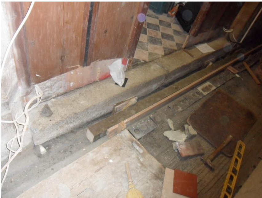
THE PIECES OF GRANITE BACK IN PLACE ON THEIR NEW BED, THE STEP IS NOW LEVEL.
