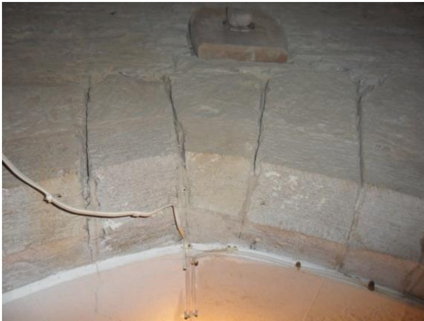
ARCH BETWEEN TOWER AND NAVE ON THE TOWER SIDE
