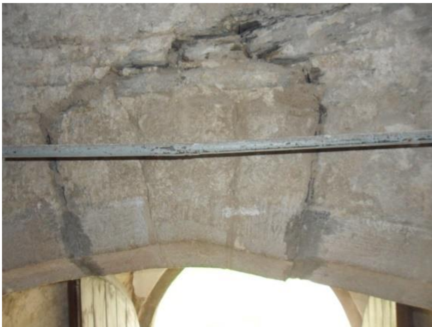
ARCH ABOVE TOWER WEST DOOR
