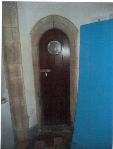
DOOR TO TOWER STAIRS OUTER LAYER REMOVED, ORIGINAL DOOR RESTORED AND REHUNG
