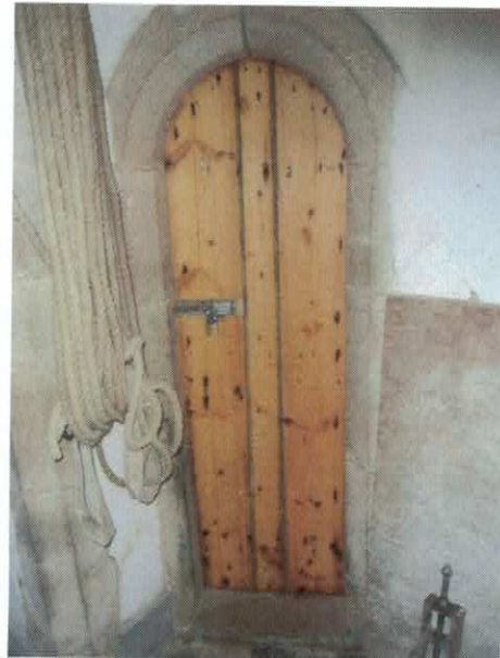
DOOR TO TOWER STAIRS OUTER LAYER REMOVED, ORIGINAL DOOR RESTORED AND REHUNG
