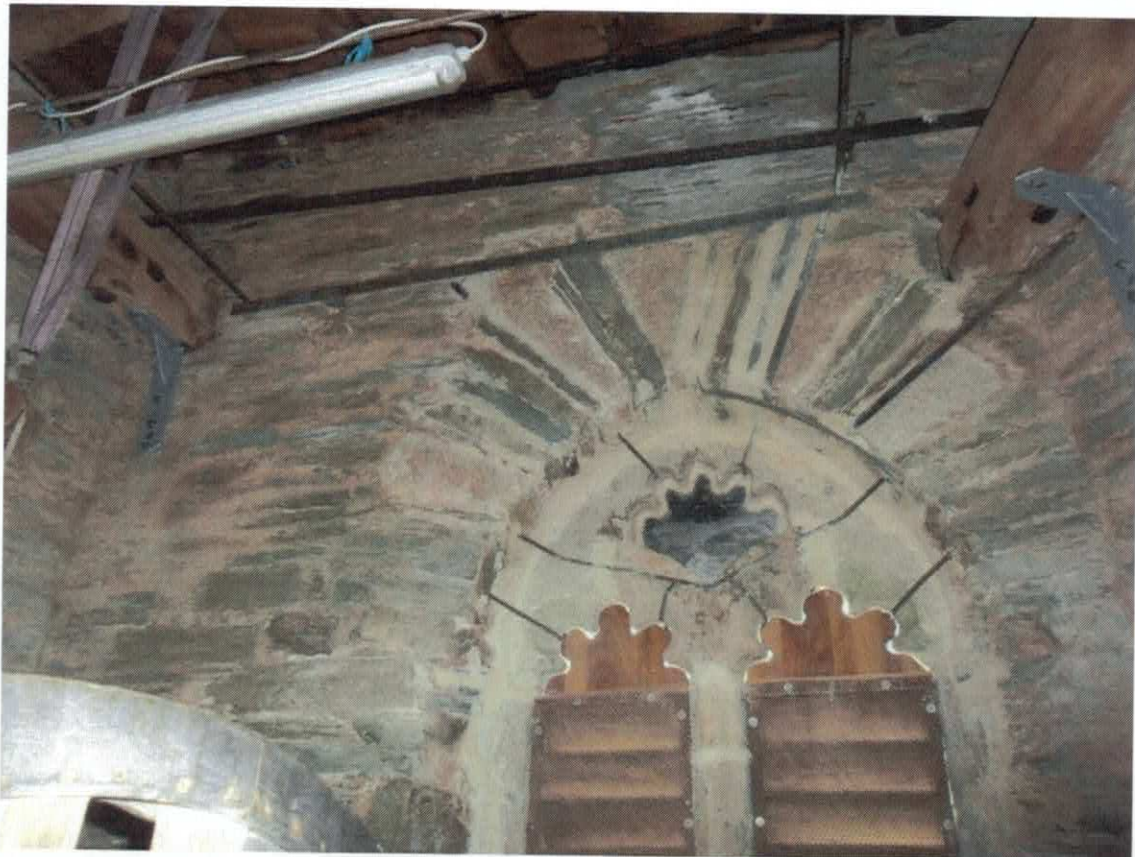
WEST BELL CHAMBER WALL INTERNAL VIEW
