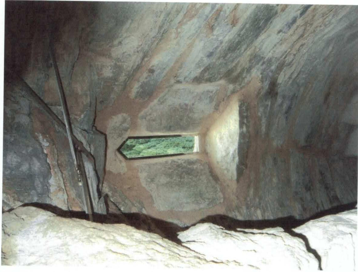
STAIR WINDOW AND CRACKED LINTEL AFTER REPAIR
