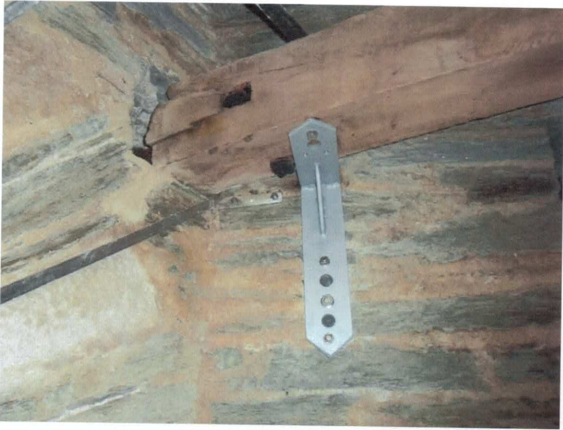
NEW BRACKET TO WEST END OF NORTHERN TIE BEAM
