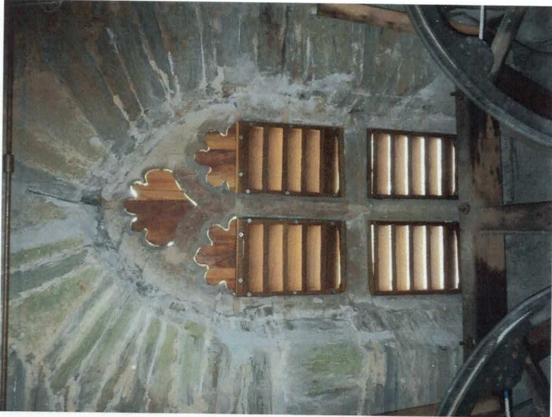
PEARSON LUBBOCK ARCHITECTS BELL CHAMBER OPENINGS BEFORE AND AFTER FIRST PHASE
