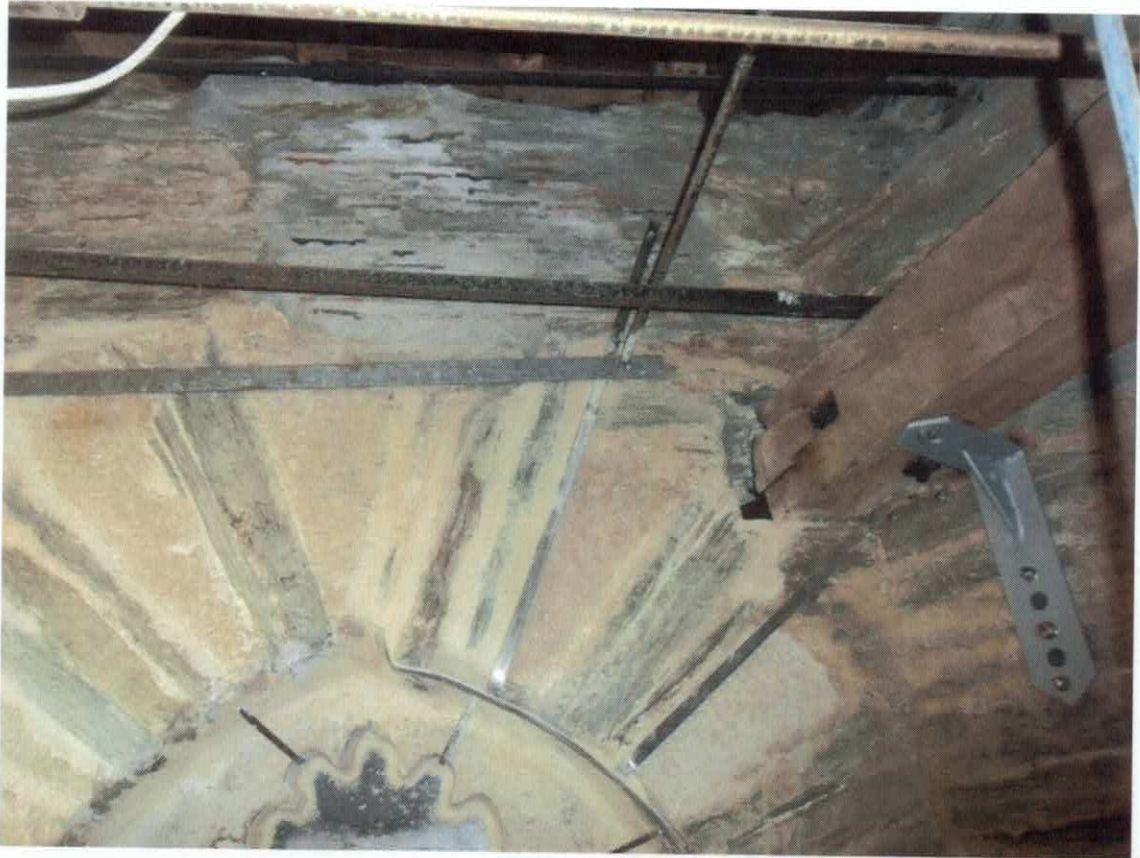
BELL CHAMBER WEST WALL AFTER REPAIR
