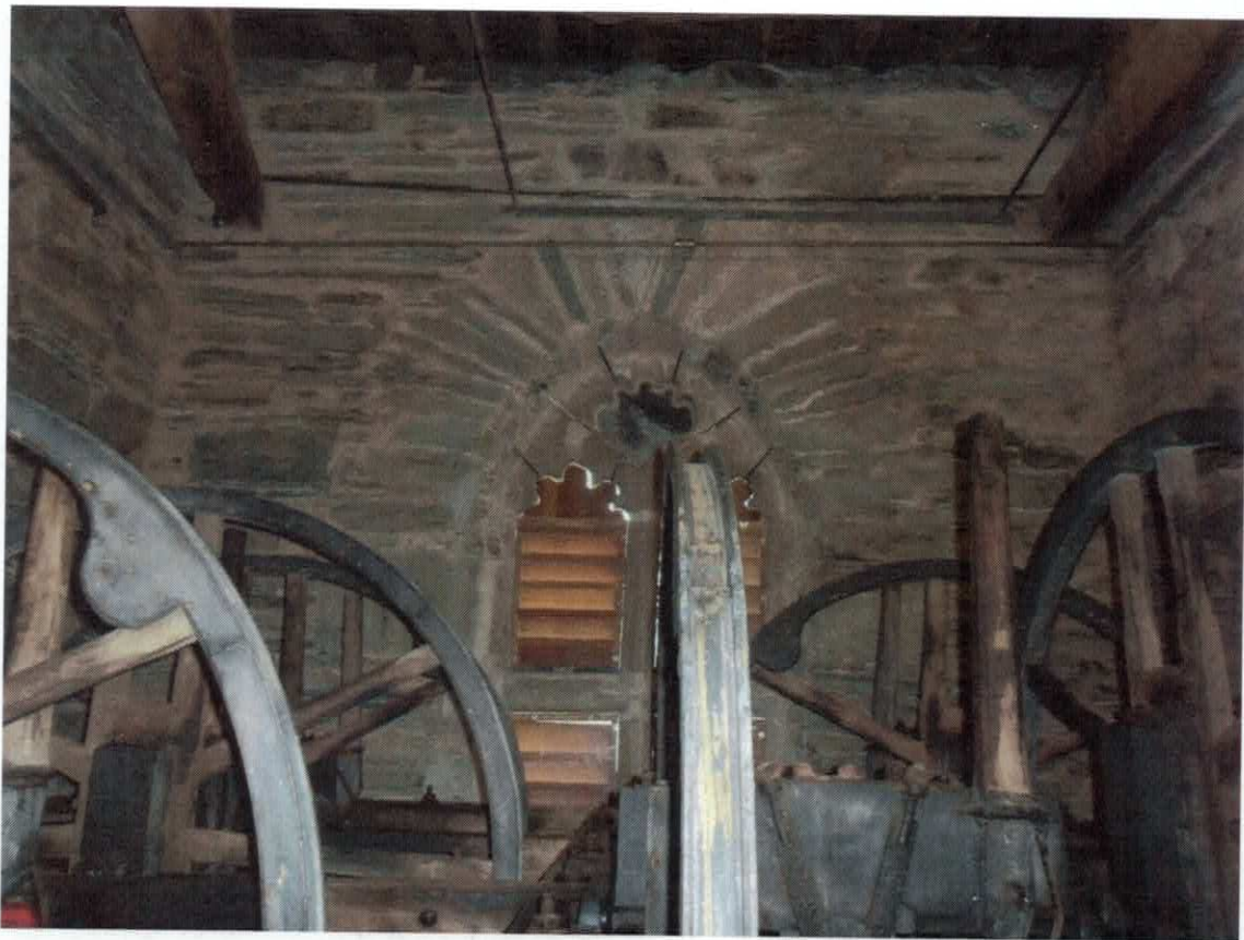
EAST BELL CHAMBER WALL INTERNAL VIEW
