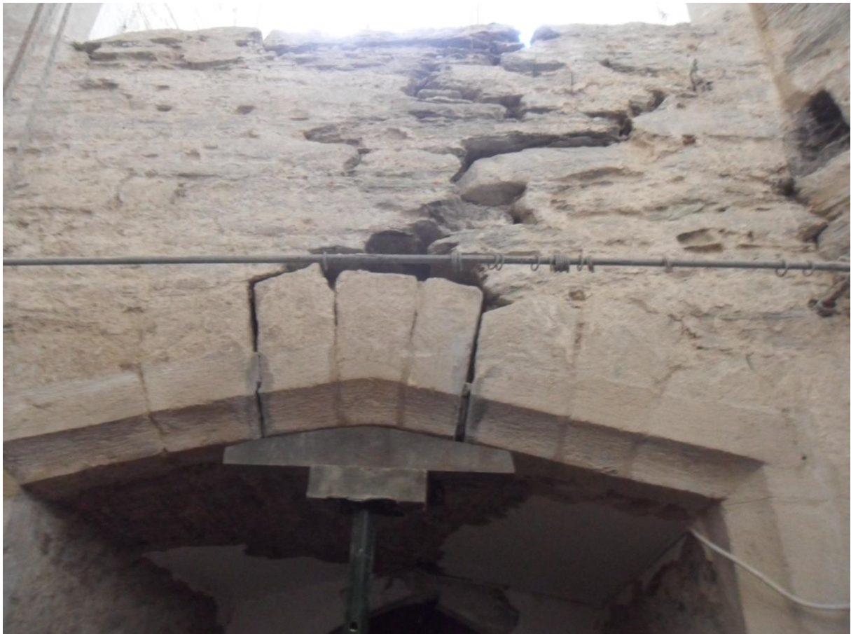
KEY STONES TO TOWER WEST DOOR ARCH HAD DROPPED
