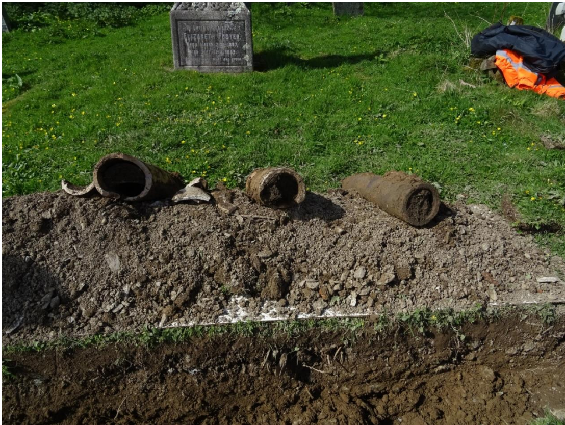
RAINWATER DRAINE FROM TOWER – BLOCKED AND BROKEN CLAY PIPES SETTLED TO IN AN UNEVEN FALL
