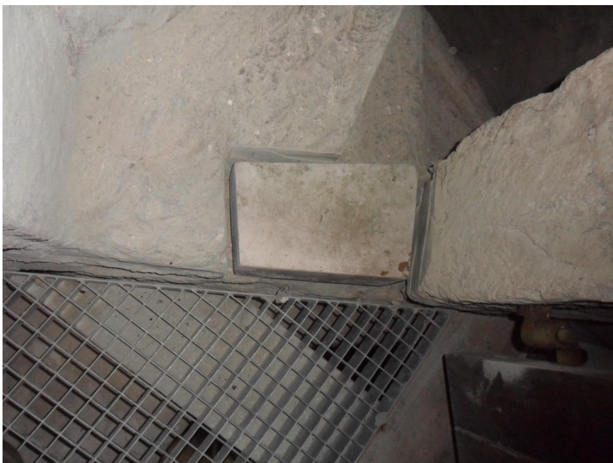
STEP TO OLD BELL CHAMBER FROM TOWER STAIR REPAIRED WITH NEW STONE
