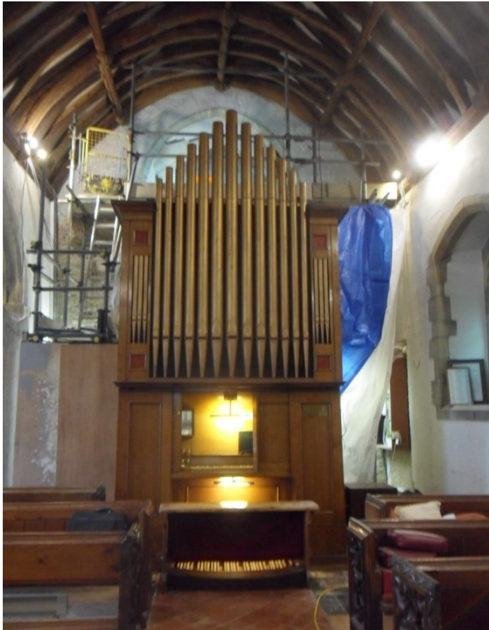
SCAFFOLD BEHIND THE ORGAN TO REPAIR THE ARCH AND REMOVE THE CEMENT RENDER
